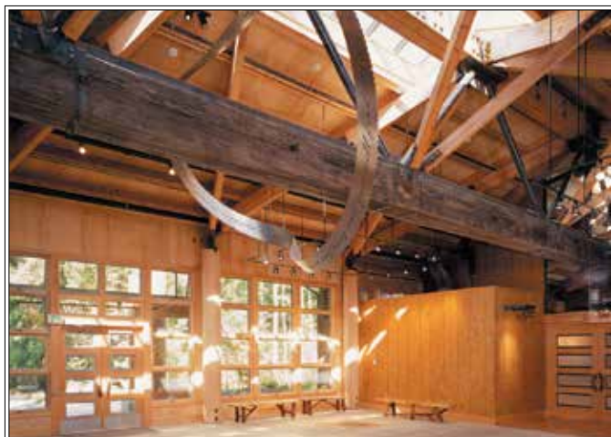
Islandwood Environmental Learning Center (LEED Gold)
