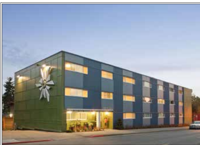
Holiday Apartments Renovation
