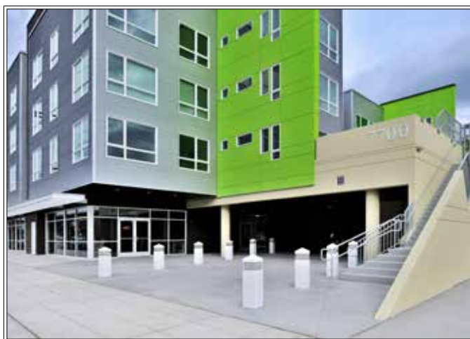
Emerald City Commons Apartments (ESDS / Built Green / Built Smart)
