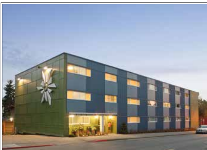
Holiday Apartments Renovation
